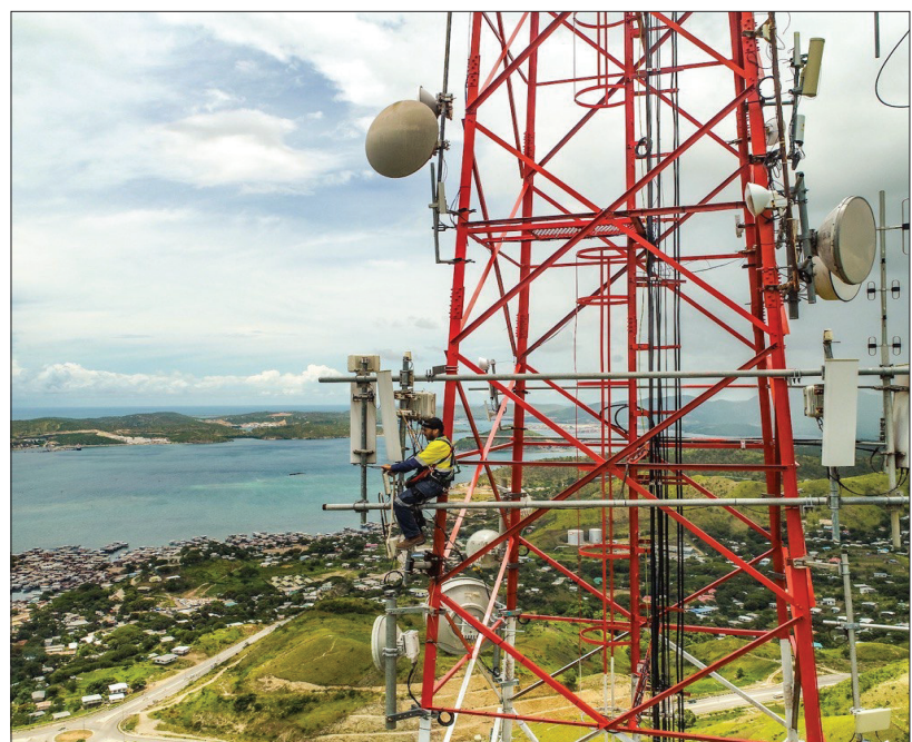
Alex Roalakana Junior conducting preventive maintenance on the Kinect LTE antenna at the Burns Peak Tower, in Port Moresby.
